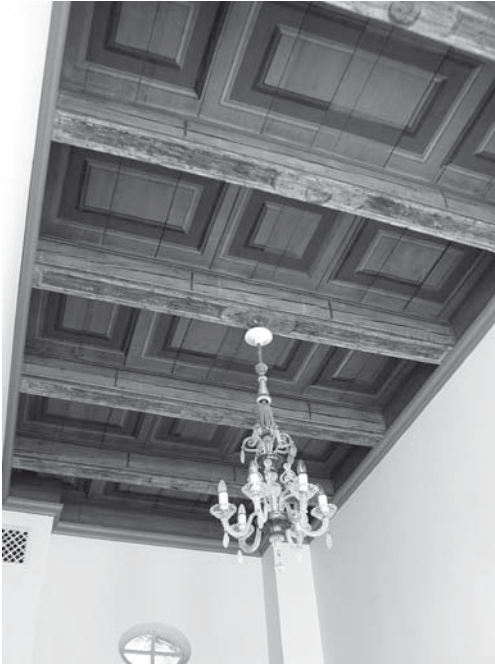
Fig. 3.B.3 Wooden ceiling with painted panel imitations, c.1655, room 1.12, Johan de Witt House in The Hague.
